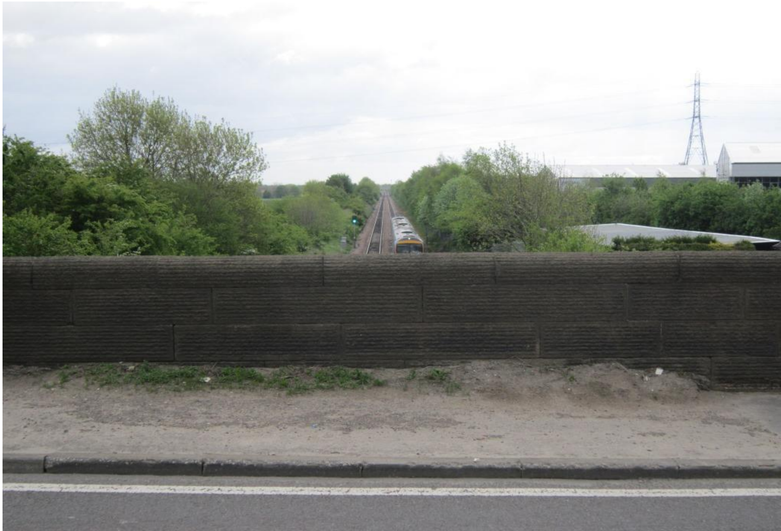
Railway Bridge over Leeds to York/Hull lines – looking east
