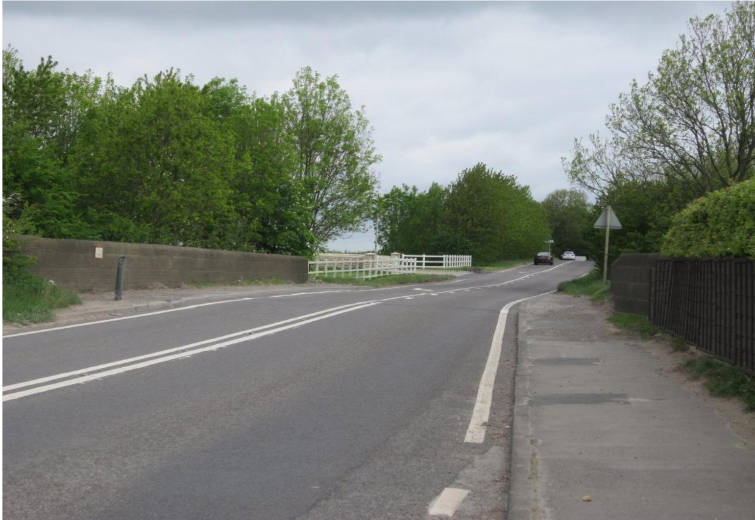
Railway Bridge over Leeds to York/Hull lines
