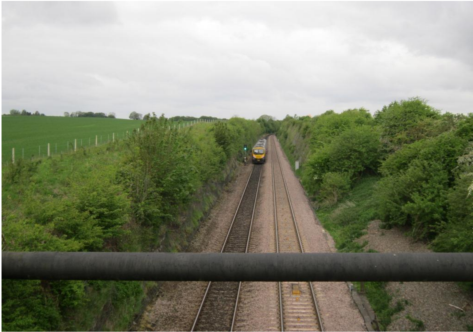
Railway Bridge over Leeds to York/Hull lines – looking west towards Garforth
