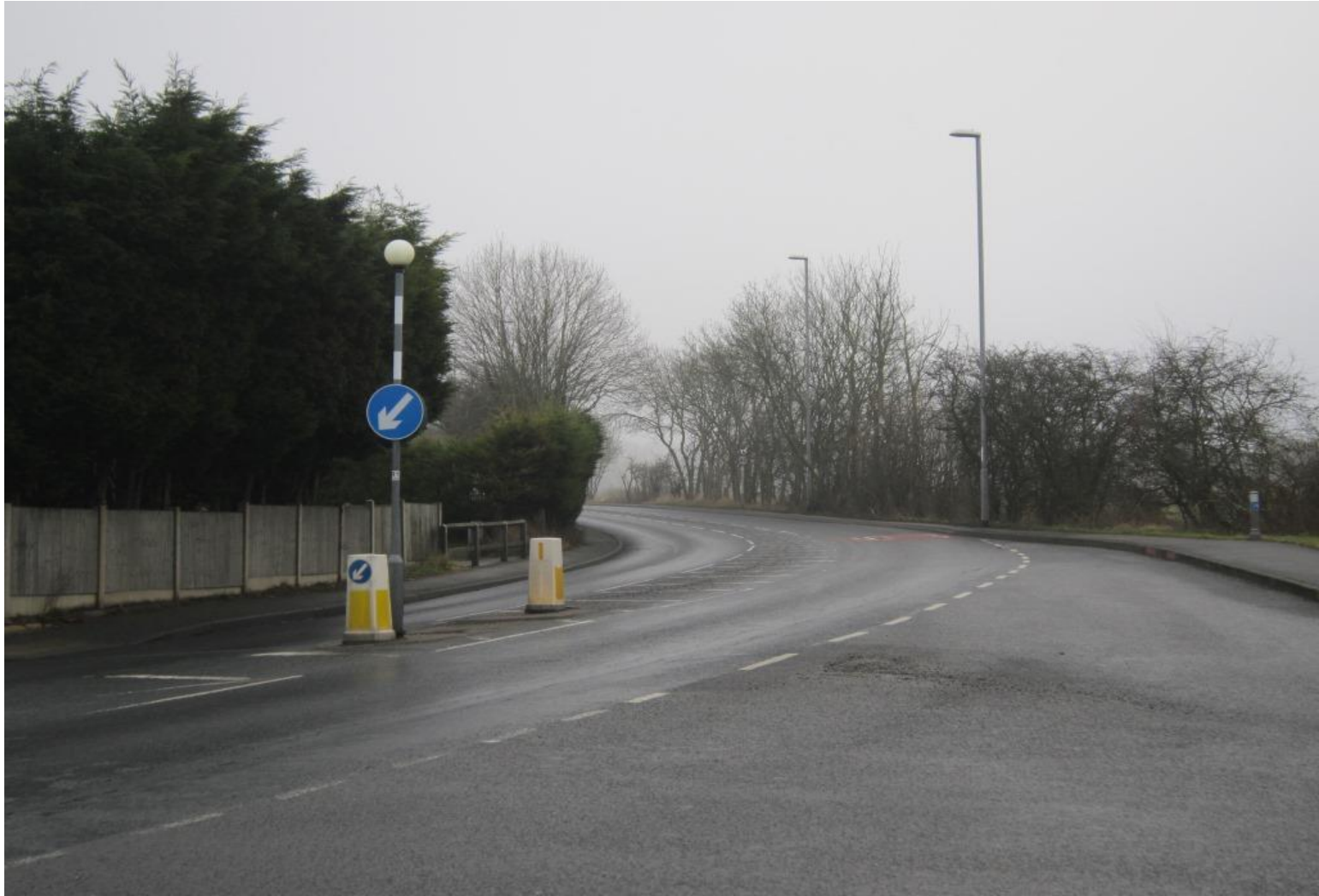
Dangerous Kippax Junction – known as Charlie Sweep's Corner
