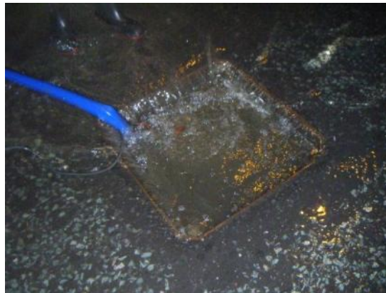
Figure 16: FRM Contractors pump Leeds Road flood into adjacent flood plain to reopen road, Friday evening, August 8 th
