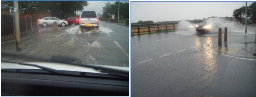
Figure 11: Leeds Road flooding at junction with Doctors Lane, Allerton Bywater
