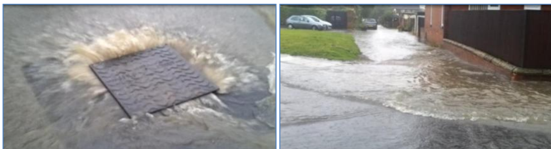
Figure 28: Surcharged culvert, flood water pathway following line of the culvert overland & downhill towards Kingsway and the Alandales
