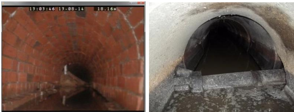
Figure 30: Photograph showing new lamp column installed through the culvert main line (Lidgett Lane) and service pipe through culvert (Alandale Crescent)
