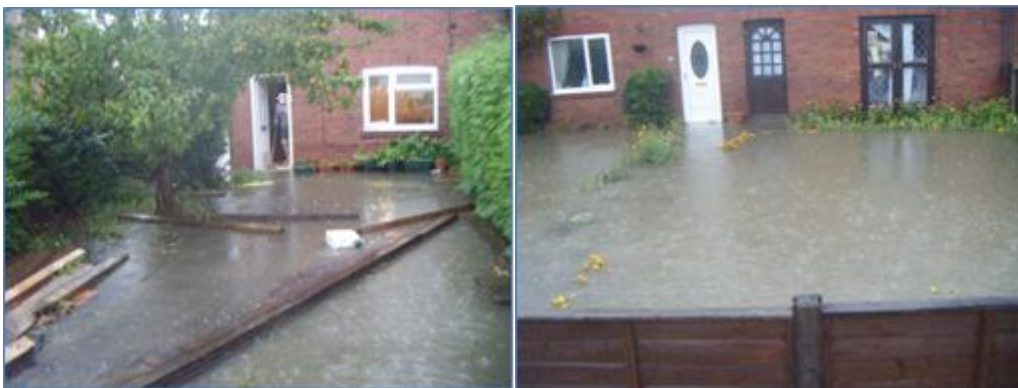
Figure 12: flooding along Leeds Road, Allerton Bywater
