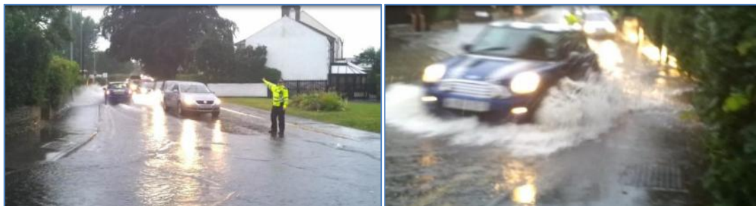
Figure 34: photographs of dangerous lake at the junction of Lowther Avenue and Lidgett Lane
